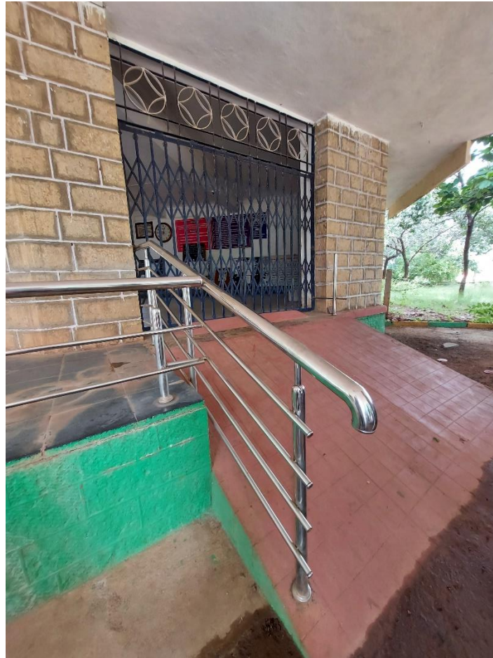
Figure 13 - Placing of ramp for use by physically challenged
